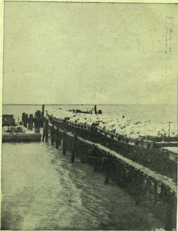
Train Loads of Rock for the Jetties.
