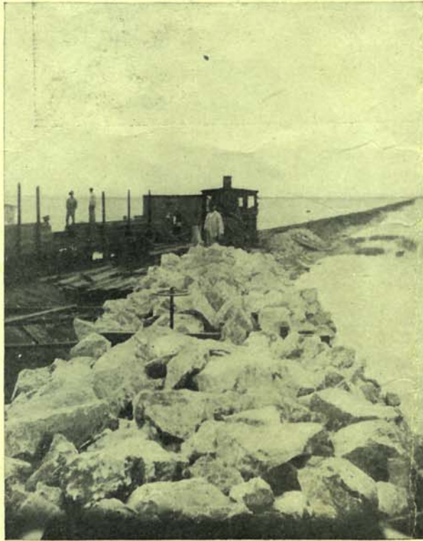
U. S. Government Work on South Jetties.
